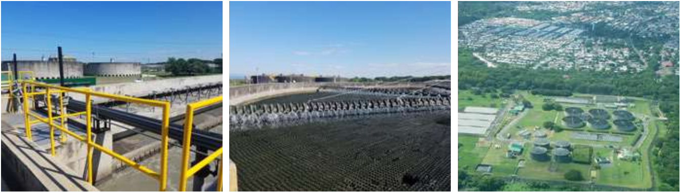
Figure 10. Managua Treatment Plant
